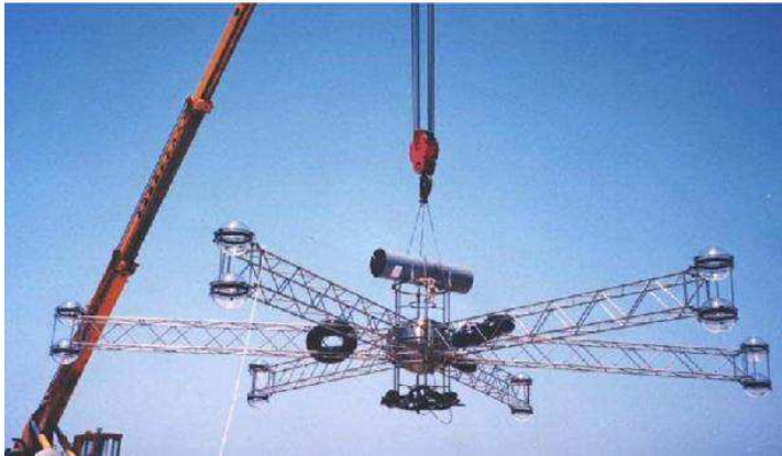
Figure 3. Reduced-size NESTOR floor during preparation for deployment.
